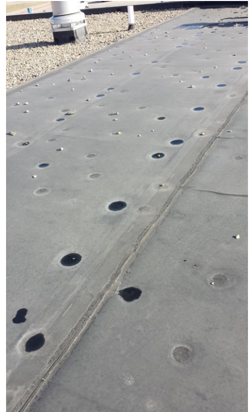
The roof of the Student Center was recently damaged by hail causing significant depressions in roof membrane.
